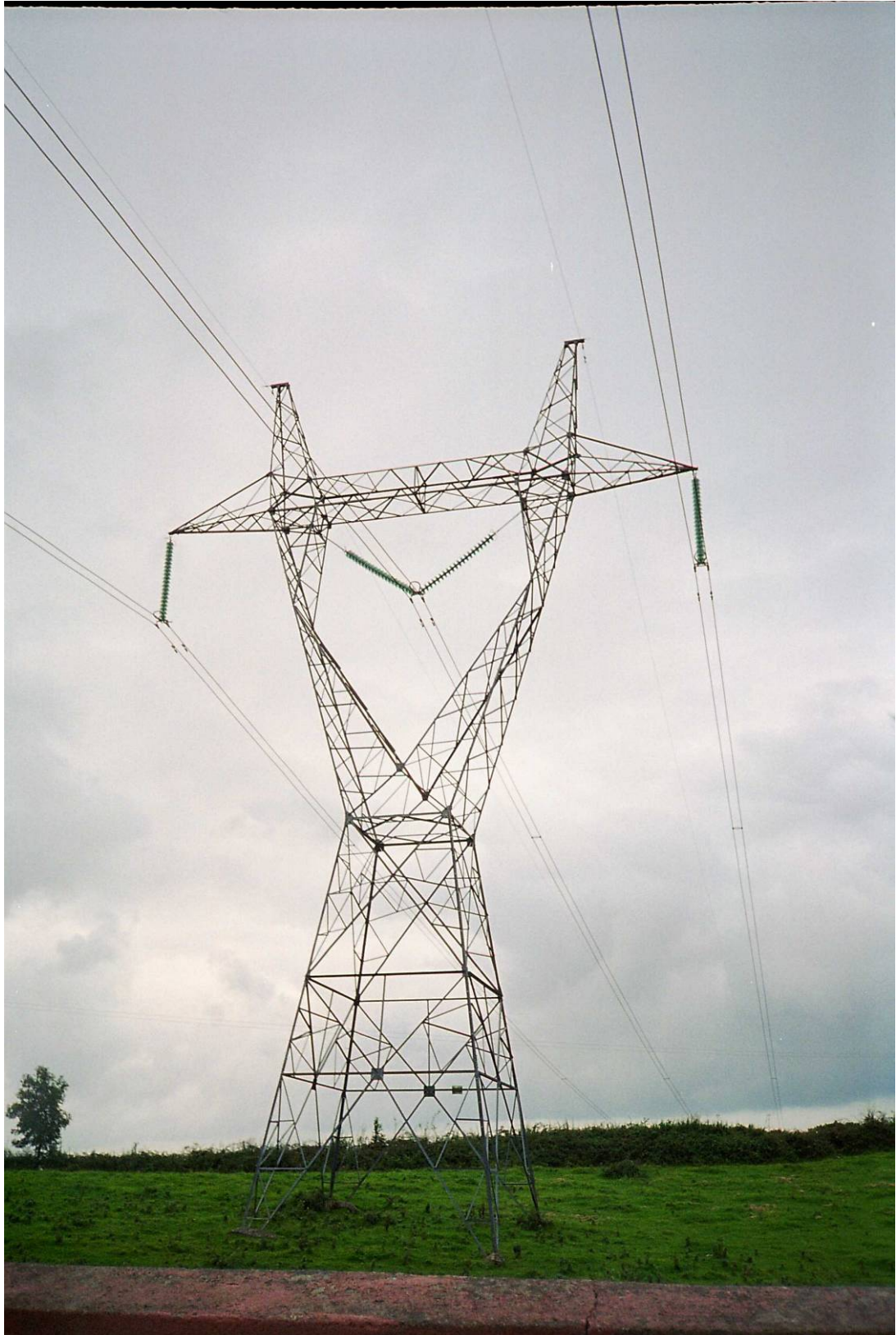
Indicative 400kV Single Circuit Intermediate Tower
